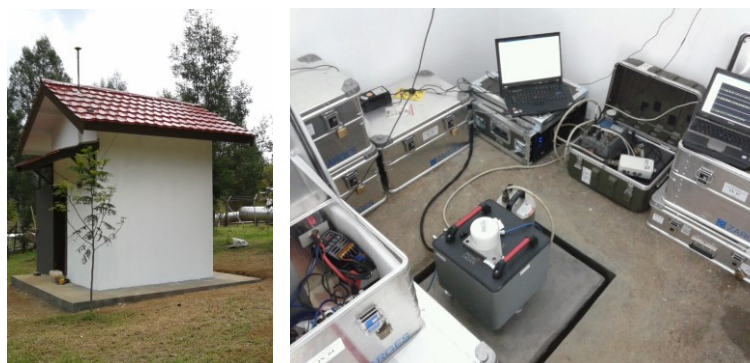
Figure 6: Gravity-meter gPhoneX 128 (right) in the specially constructed new observation building (left): the pillar of the gravity-meter is completely decoupled from the building. An additional installation of a Trillium compact seismic sensor and a tilt-meter on the pillar is used for detailed signal analysis and comparison of the gravity signal with the signals of the seismic network.
