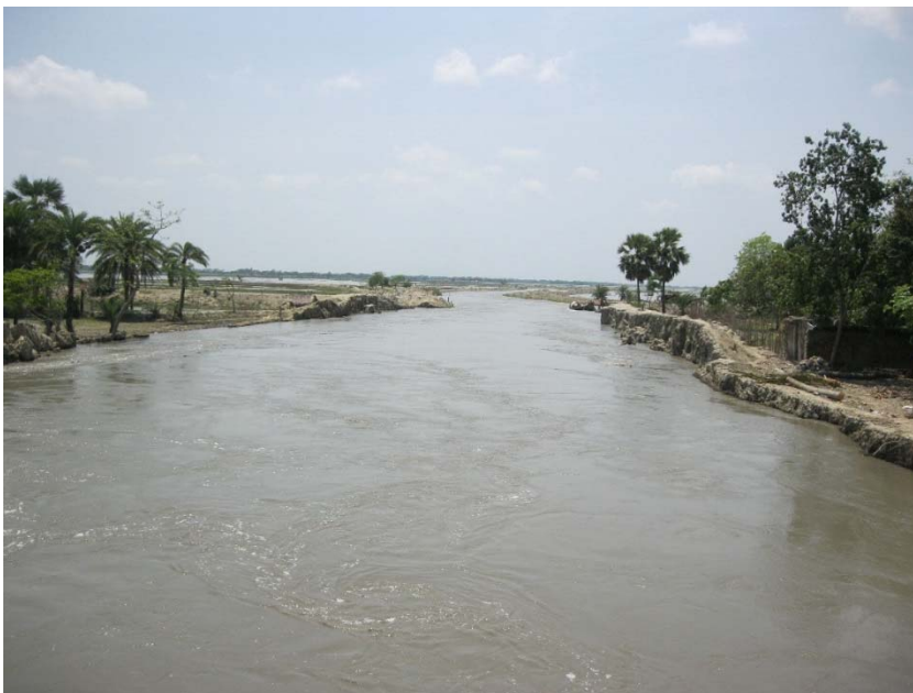
Figure 4. Ongoing TRM in Beel Pakhimara . The figure illustrates water carrying sediment entering into the floodplain from the river.
