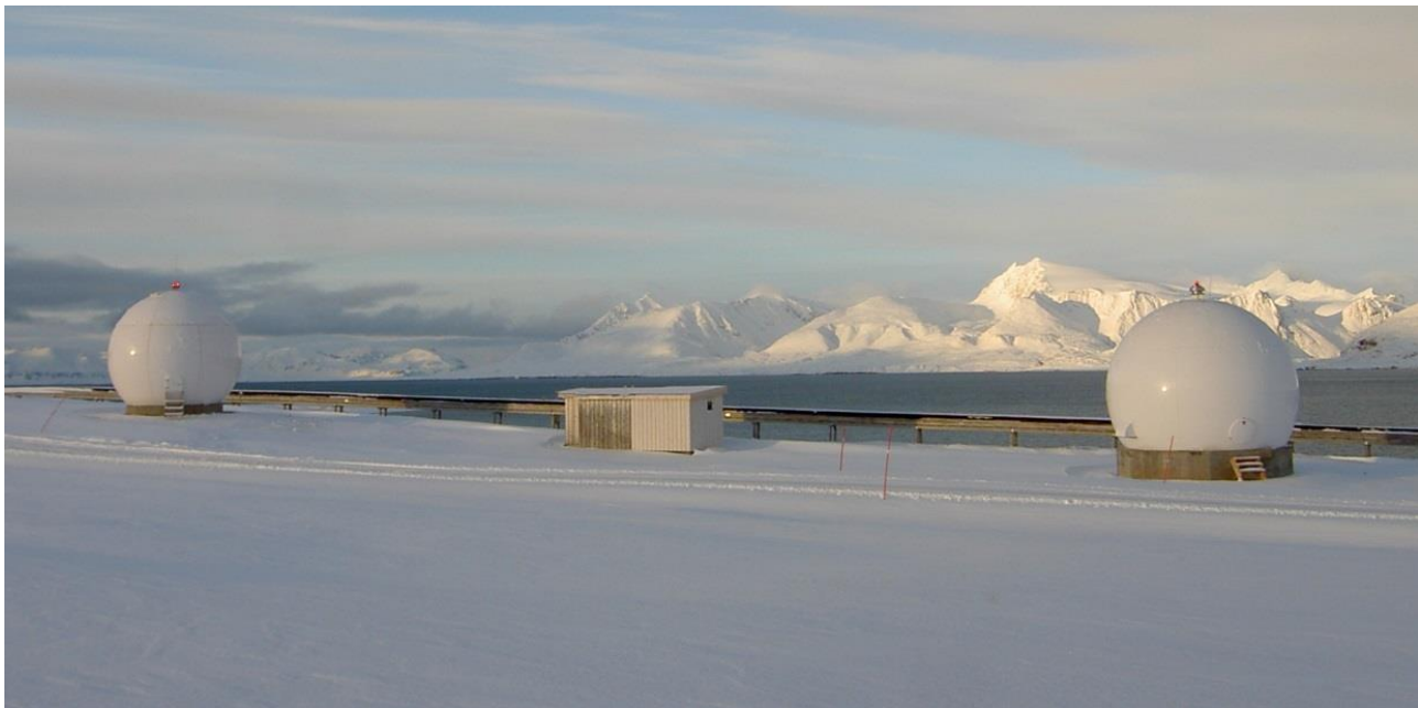
Figure 1: The satellite receiving station Ny-Ålesund with two antennas and a hut with further receiving equipment
