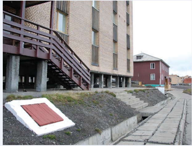
Figure 2.4 House built on pillars in Barentsburg, Svalbard. These pillars allow air circulation underneath the building to protect the permafrost (Margareta Johansson).
