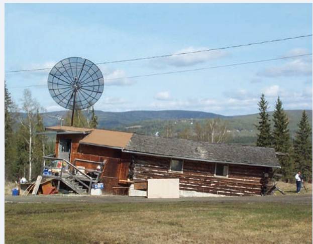
Figure 2.5 Ice in the permafrost has melted and the ground has collapsed resulting in a house that is no longer possible to live in (Vladimir Romanovsky).
