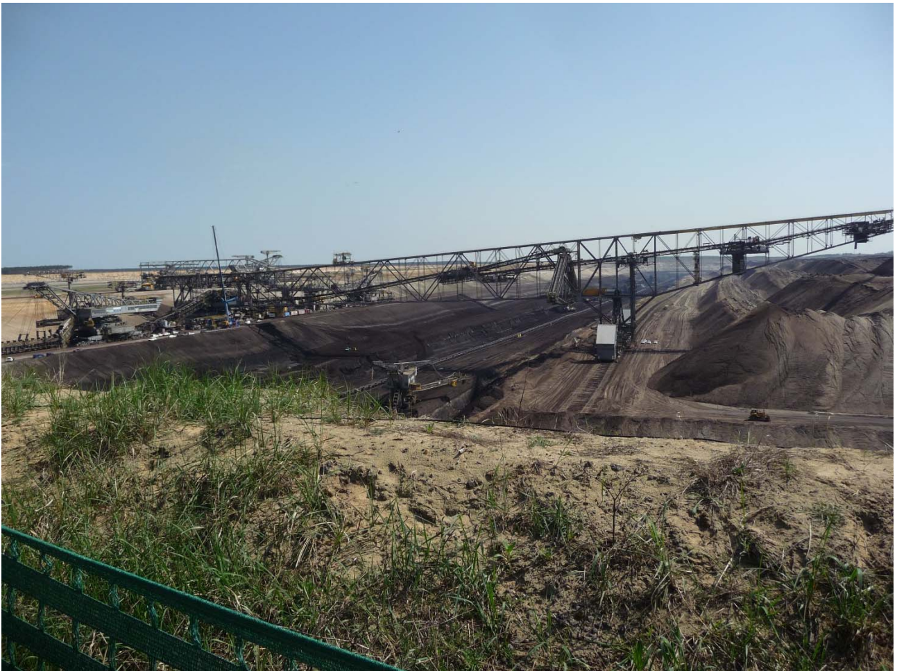
Fig. 6: View of the opencast lignite mine of Jänschwalde, with the overburden conveyer bridge. The view is to the east (photo: H. Rösler). – Figure from Raab, T. et al. (2015).
