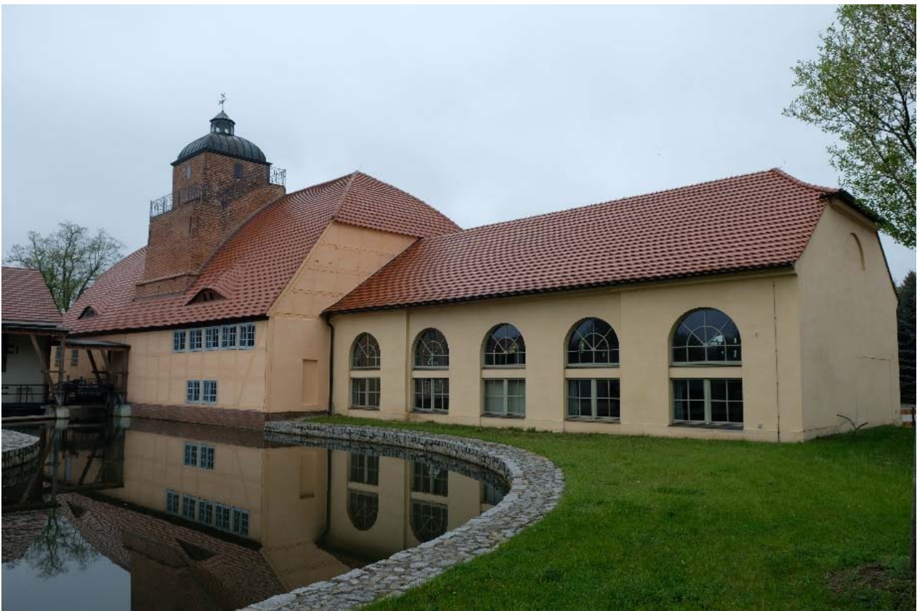
Fig. 14: Blast furnace building of the Peitz ironworks.
