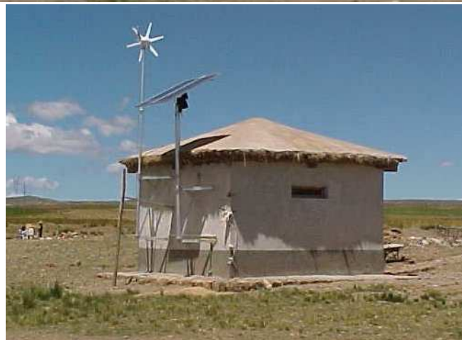
Figure 3: Observatory buildings at VRE. a) Overview over the observatory premises with a corner of the main building on the right. b) Power supply building with solar panel and wind generator.
