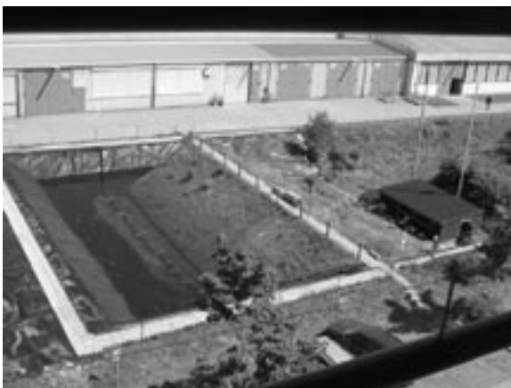
Figure 1: Aerial view of the flooded model dike at the Federal Waterways and Research Institute in Karlsruhe
