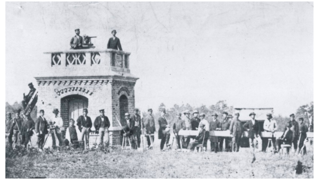
Figure 4. Baseline measurement in Großenhain in 1872, western end point at Raschütz, Nagel (left) and Helmert on the observation building (unknown source).
