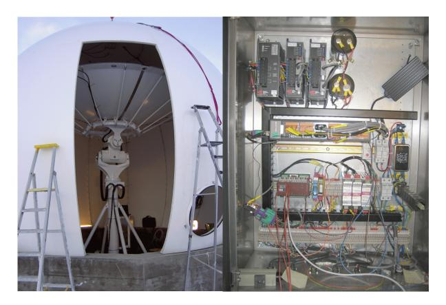
Figure 44: NYA-2 antenna system and servo control cabinet
