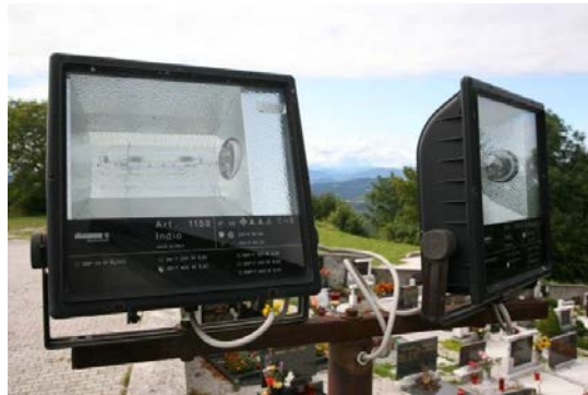
Figure 2: The two 400-Watt metal-halide reflector floodlamps used in the original lighting.
