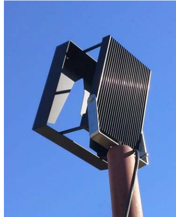
Figure 5: Photo of an EcoSky LED with mask for the Church of the Three Kings in place.
