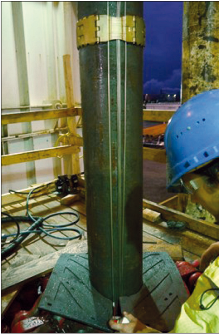
Fig. 3 Installation of fiber optic cable behind 9 5/8" casing in IDDP-2 well (Foto: Martin Lipus, GFZ)
