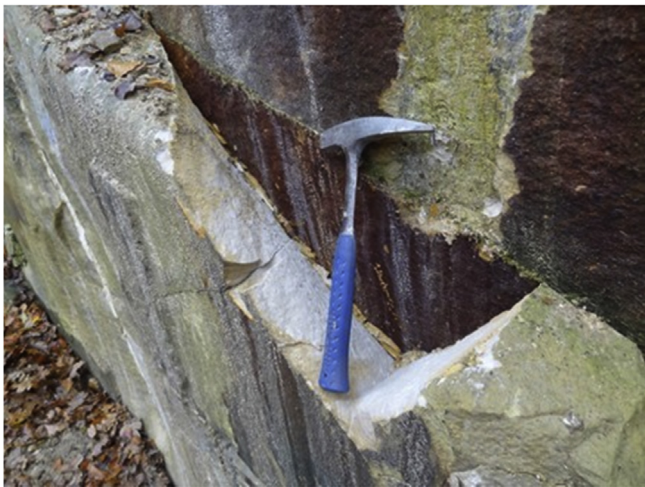
Fig. 2. Fracture face in Gildehaus quarry. Reddish-brown colours originate from iron–manganese minerals.
