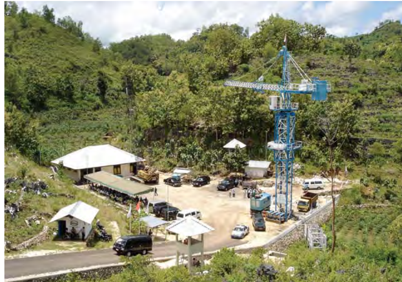
Drill site in the karst area
