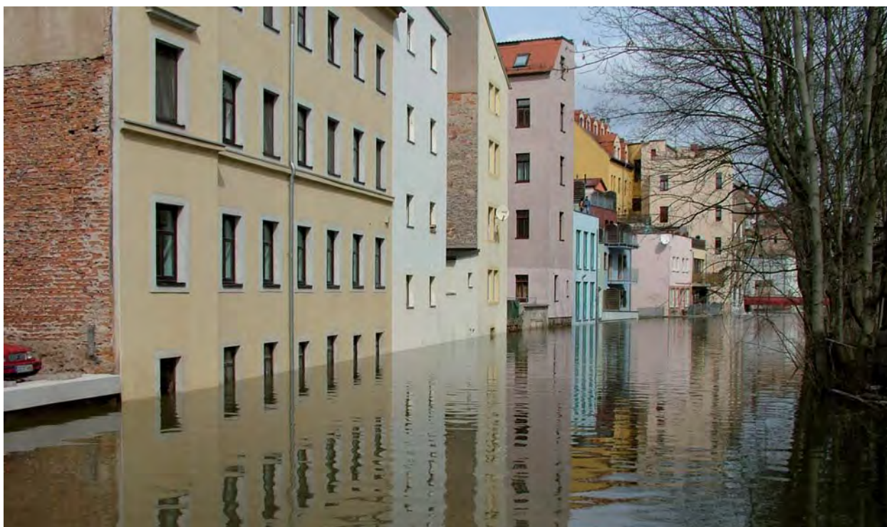
Threat from below: groundwater escaping to the surface
