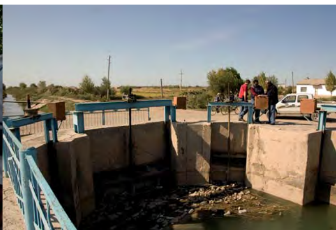
An irrigation channel with distribution structure
