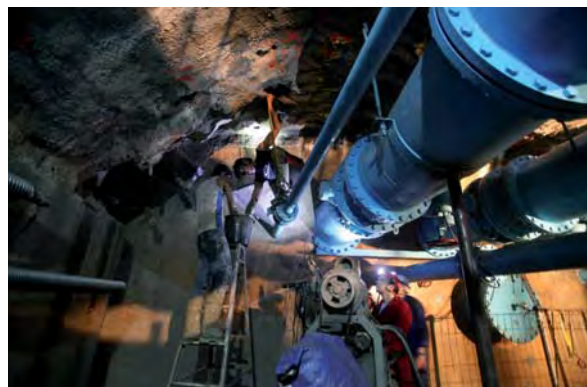
Construction work in the cave
