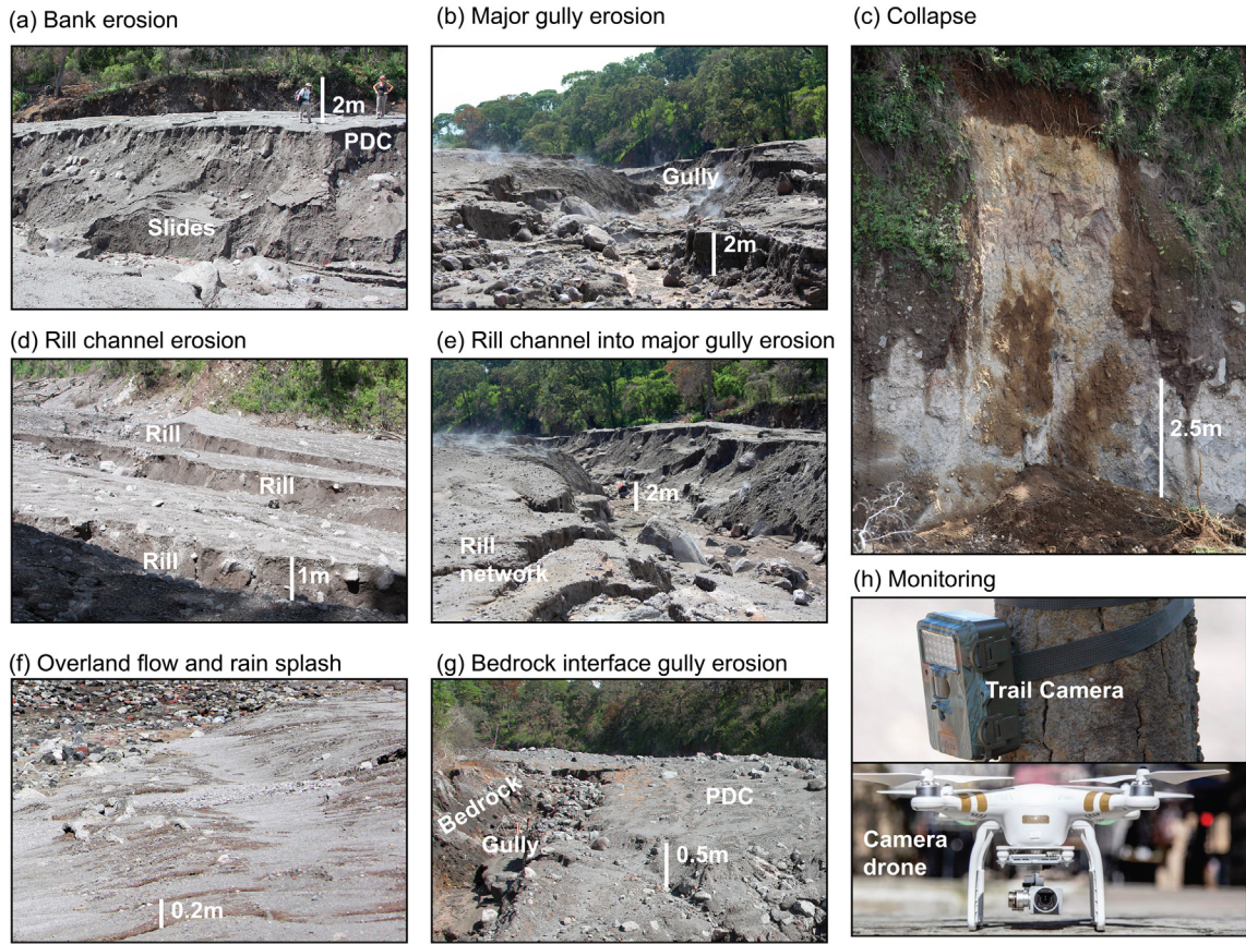
Fig. 3. (a) Field photographs illustrating different types of erosion in the Montegrande valley (a–g) and the camera devices used for monitoring geomorphological changes (h). See text for more details.
