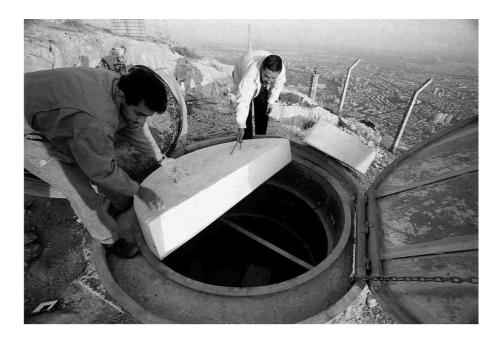
**Fig. 7.42** Installing thermal cover in a seismic vault. In climates with large diurnal temperature changes the cover should be positioned lower in the vault where external ground temperature does not change significantly.
