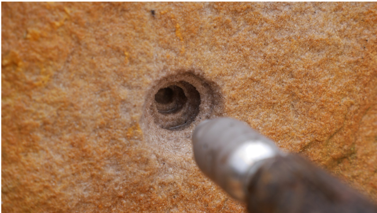
figure 9: jetted borehole in Bad Bentheim/Gildehaus sandstone with rotating nozzle design
