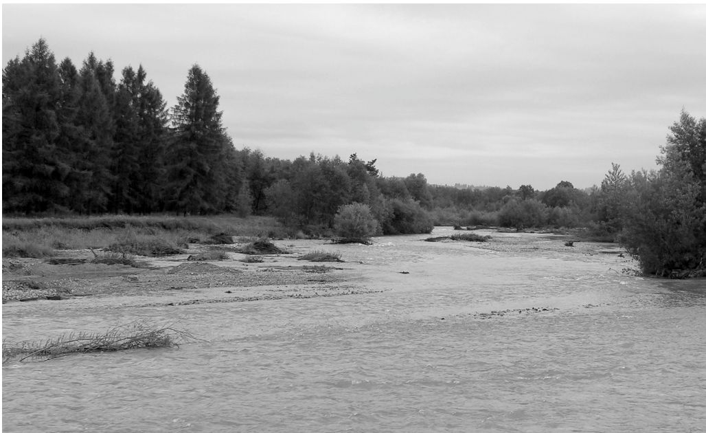
Figure 2: A section of the Czarny Dunajec River channelized in the mid-1970s (photo taken in 2012). The single-thread channel, about 40 m wide and with banks 2.4-2.6 m in height, is the result of the channelization and subsequent channel incision. The investigated riparian forest consists of the introduced European larch (higher trees) and grey alder typical of the riparian habitat.
