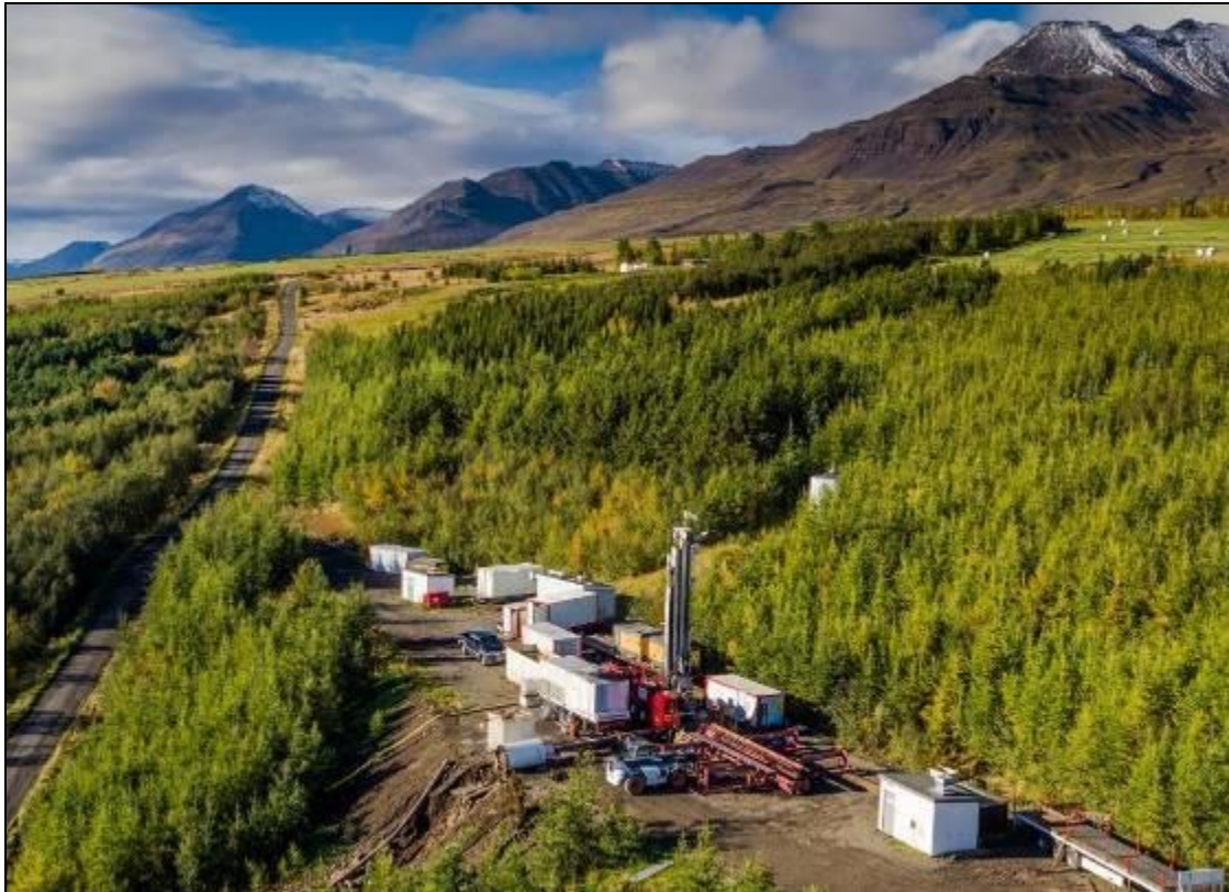
Figure 12. Drillrig Nasi on well HN-13 on September 23 rd 2016 (Photo: Auðunn Níelsson)
