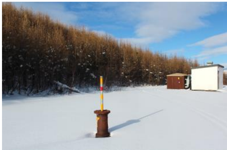
Figure 17. Well HN-13 closed and without wellhead pressure. House of well HG-10 is seen in background about 20 m away. Picture taken in March 2018 (Picture: ÍSOR/GSK).
