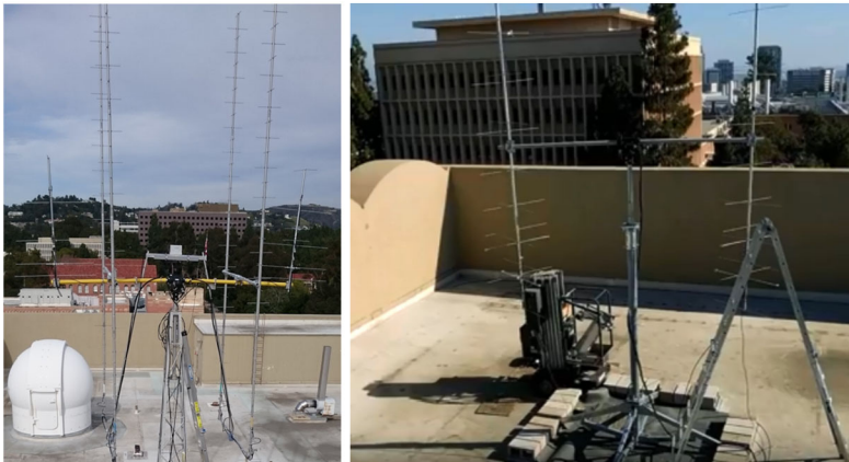
Fig. 17 Left: UCLA's Knudsen North station with four UHF yagi antennas (downlink) and two VHF yagis (uplink, using power 10 W). The spacing between UHF antennas is 6 feet on each side, and the spacing between VHF antennas is 10 feet. Right: Knudsen South station is a two VHF yagi providing higher output power (100 W). Both stations can be used simultaneously and provide flexibility when both ELFIN satellites are within view
