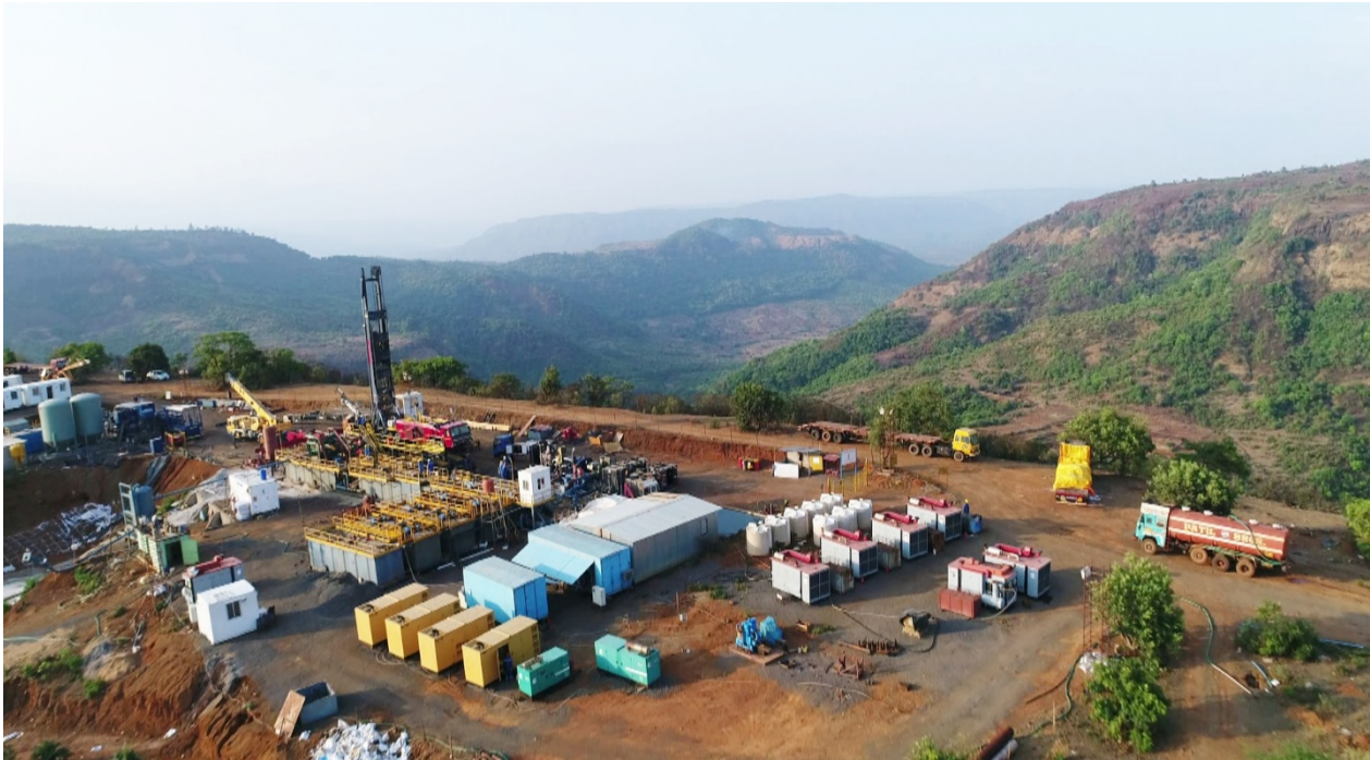
Figure 2: Drilling the 3 km deep Koyna/India pilot hole for near field studies of reservoir-triggered earthquakes.
