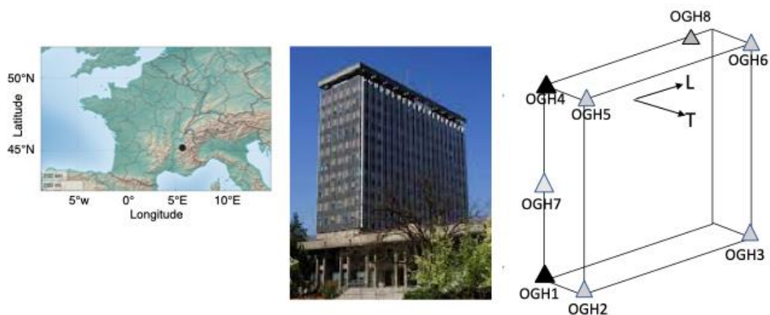
Figure 23 View of the city hall building in Grenoble and description of the monitoring array. The two stations highlighted in black (OGH1 and OGH4) are those used in this study.
