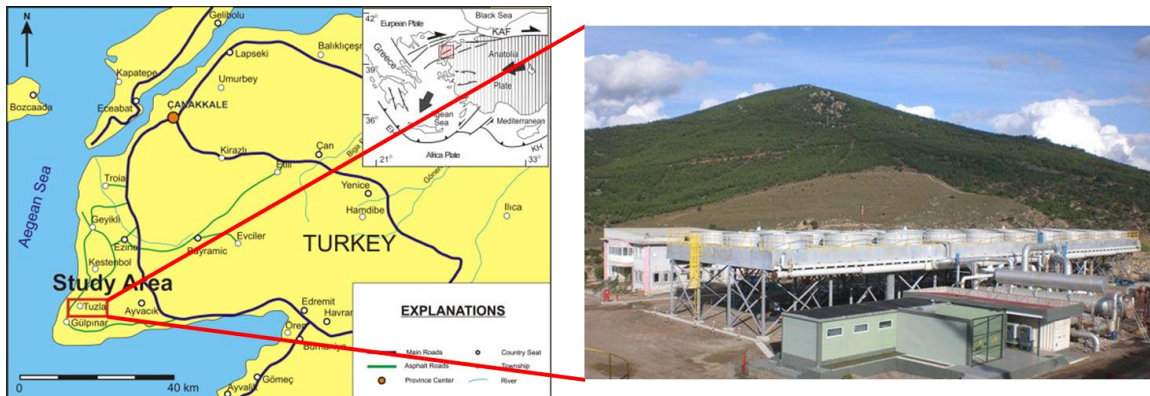
Figure 5.1. Tuzla Geothermal Power Plant located in Çanakkale, Ayvacık (Türkiye).
