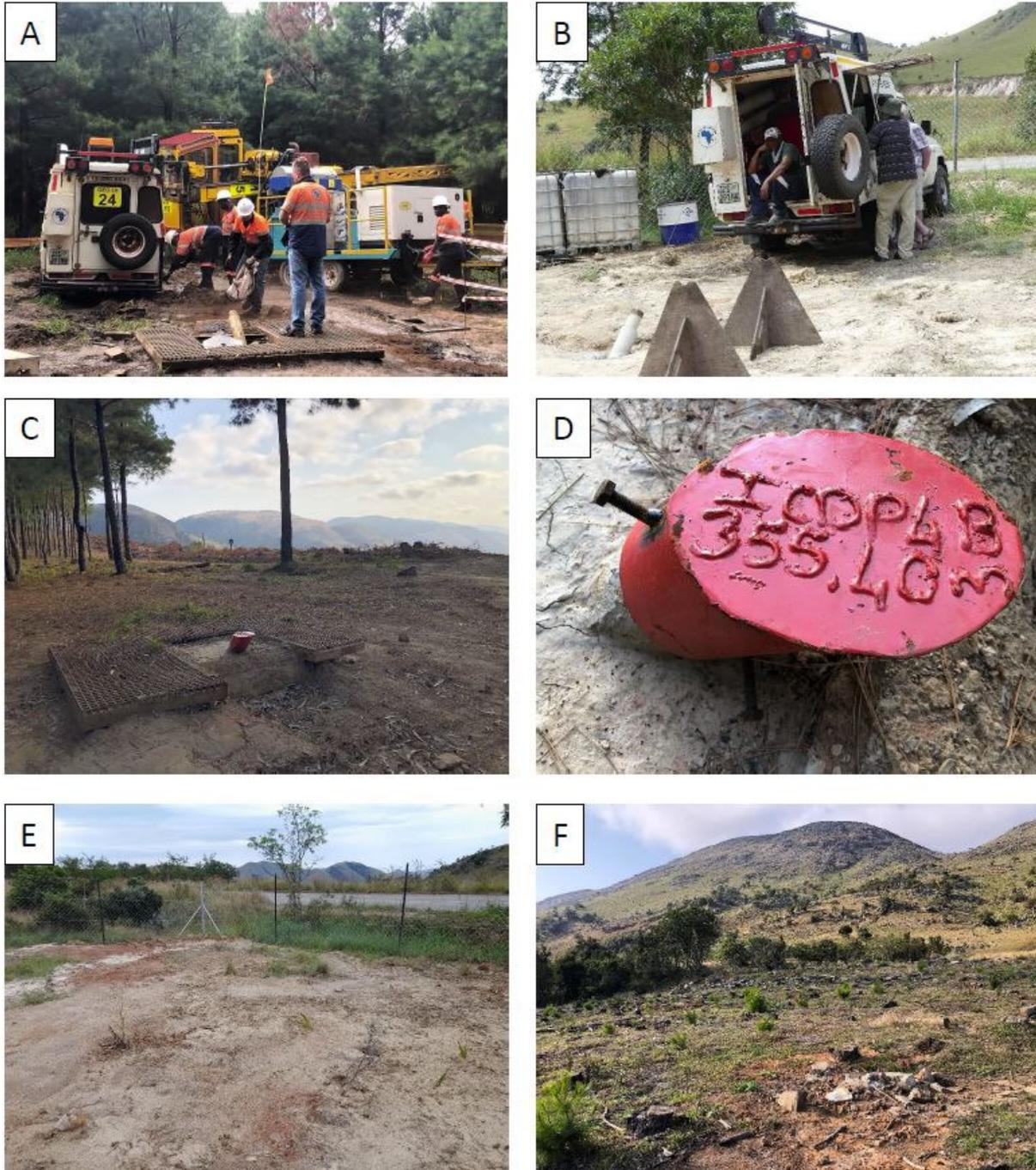
Figure 13: Post-drilling site operations. A, B: Logging; C, D: Site 4 B with cap welded on; steel grating is yet to be removed; E: Site 2 with equipment removed; site still needs to be raked and fence removed; F: Site 4C rehabilitated.
