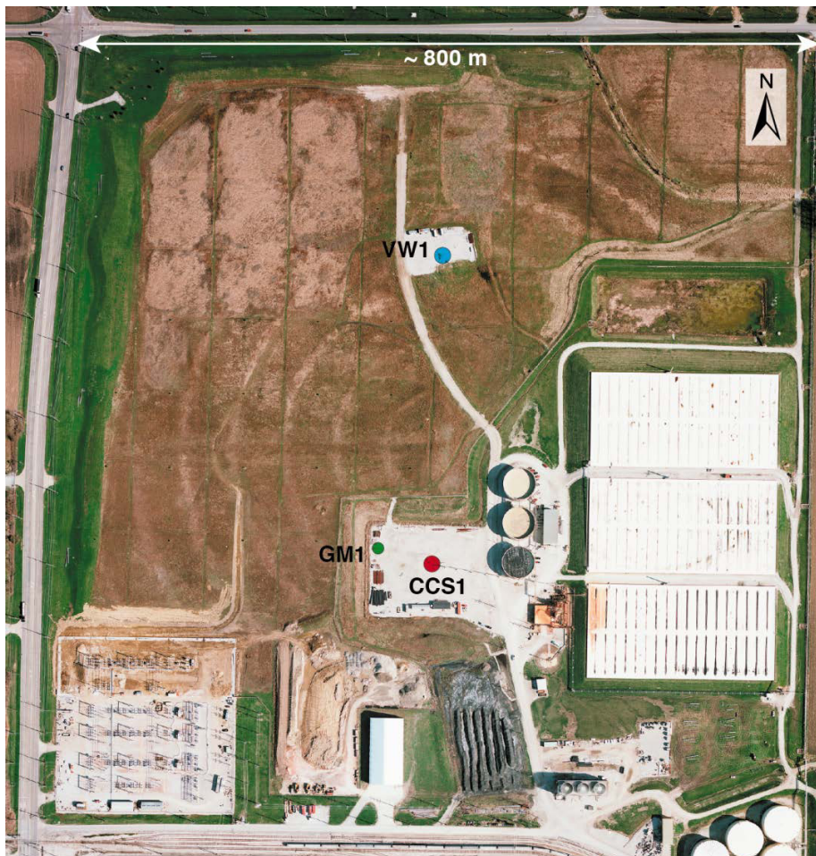
Fig. 2 IBDP pilot site: Location and aerial view with well infrastructure
