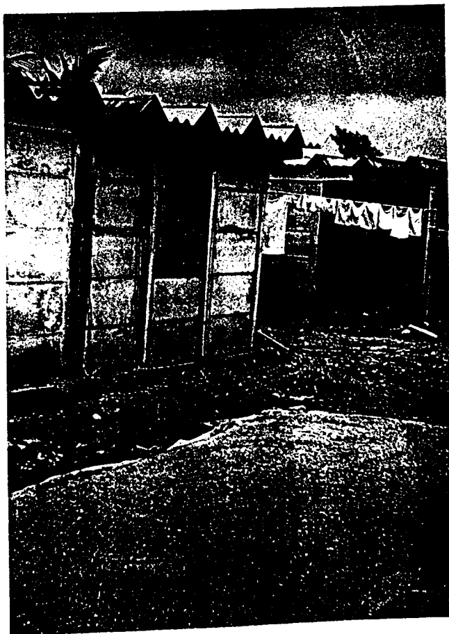
Fig. 10 Prefabricated concrete panel system type "Sandino"
