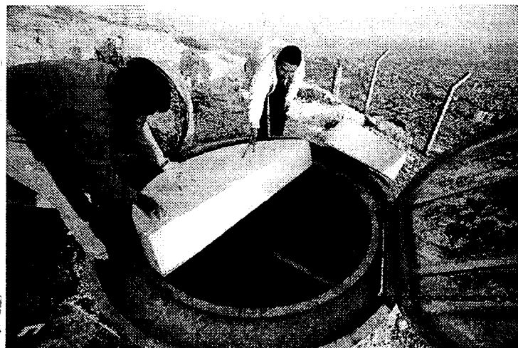
Fig. 4: Installing thermal cover in a seismic vault. In climates with big diurnal temperature changes the cover should be positioned lower in the vault where external ground temperature does not change significantly.
