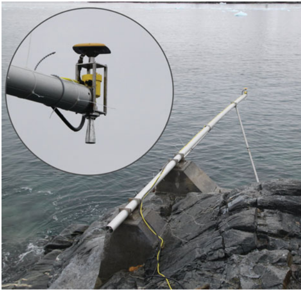
Fig. 7. (Colour online) Installation of the radar gauge system. Inset shows detail with GNSS antenna on top and radar waveguide below.
