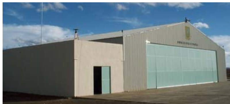
Figure 2.3: GPS station on top of side roof on hangar of Zacatecas airport.
