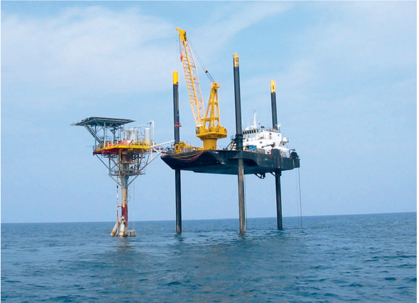
Figure 37. Jack up platform used in shallow waters inaccessible for drilling vessels and land drill rigs.
