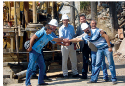
Figure 13. Start of drilling at the GONAF location in Tuzla, Turkey
