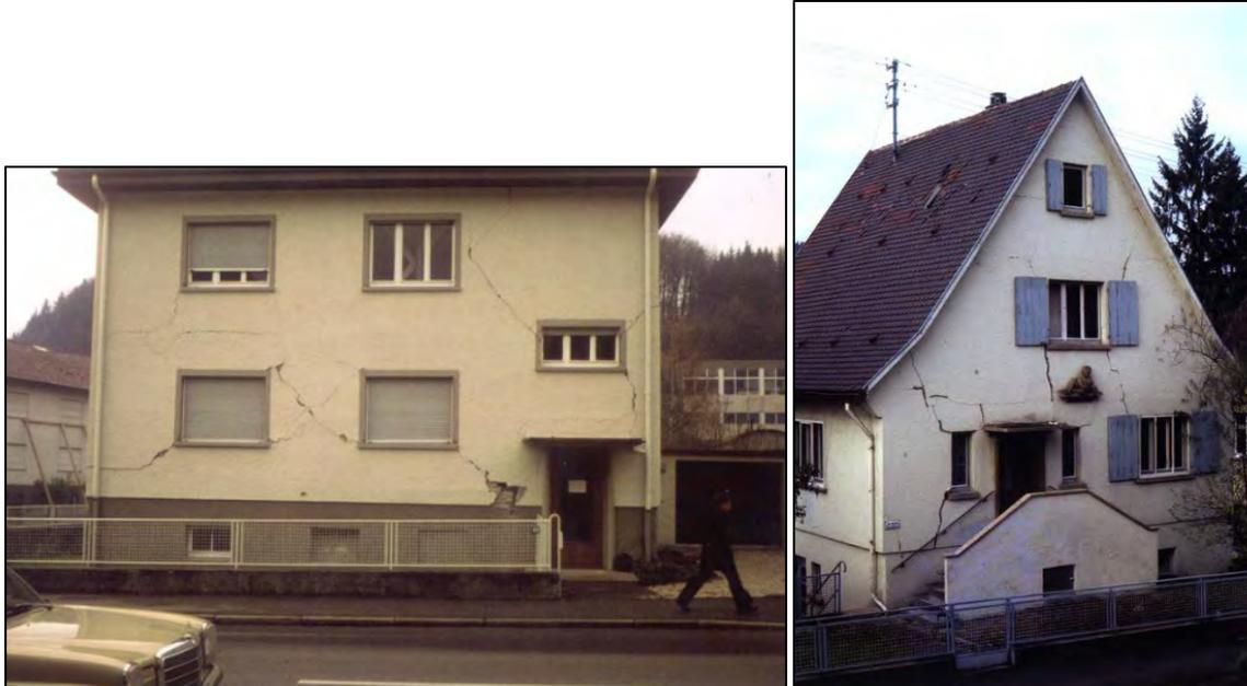
Figure 9.60: Buildings classified as suffering from EMS-98 damage grade 3 after the 1978  $M_w$  5.1 Albstadt (Baden-Württemberg) earthquake. Photos and damage assessment taken from Schwarz et al. (2010).
