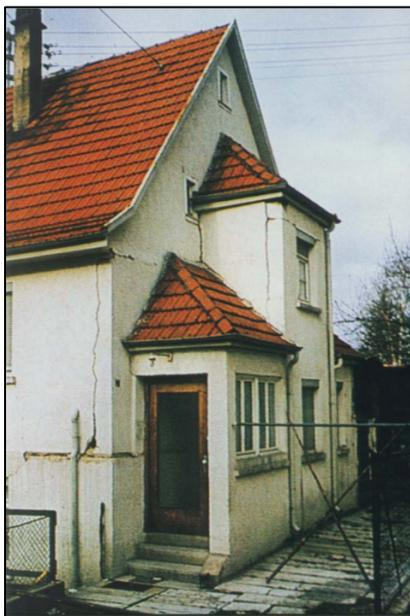
Figure 9.61: Building classified as suffering from EMS-98 damage grade 2 after the 1978  $M_w$  5.1 Albstadt earthquake. Photo and damage assessment from Grünthal (1998).
